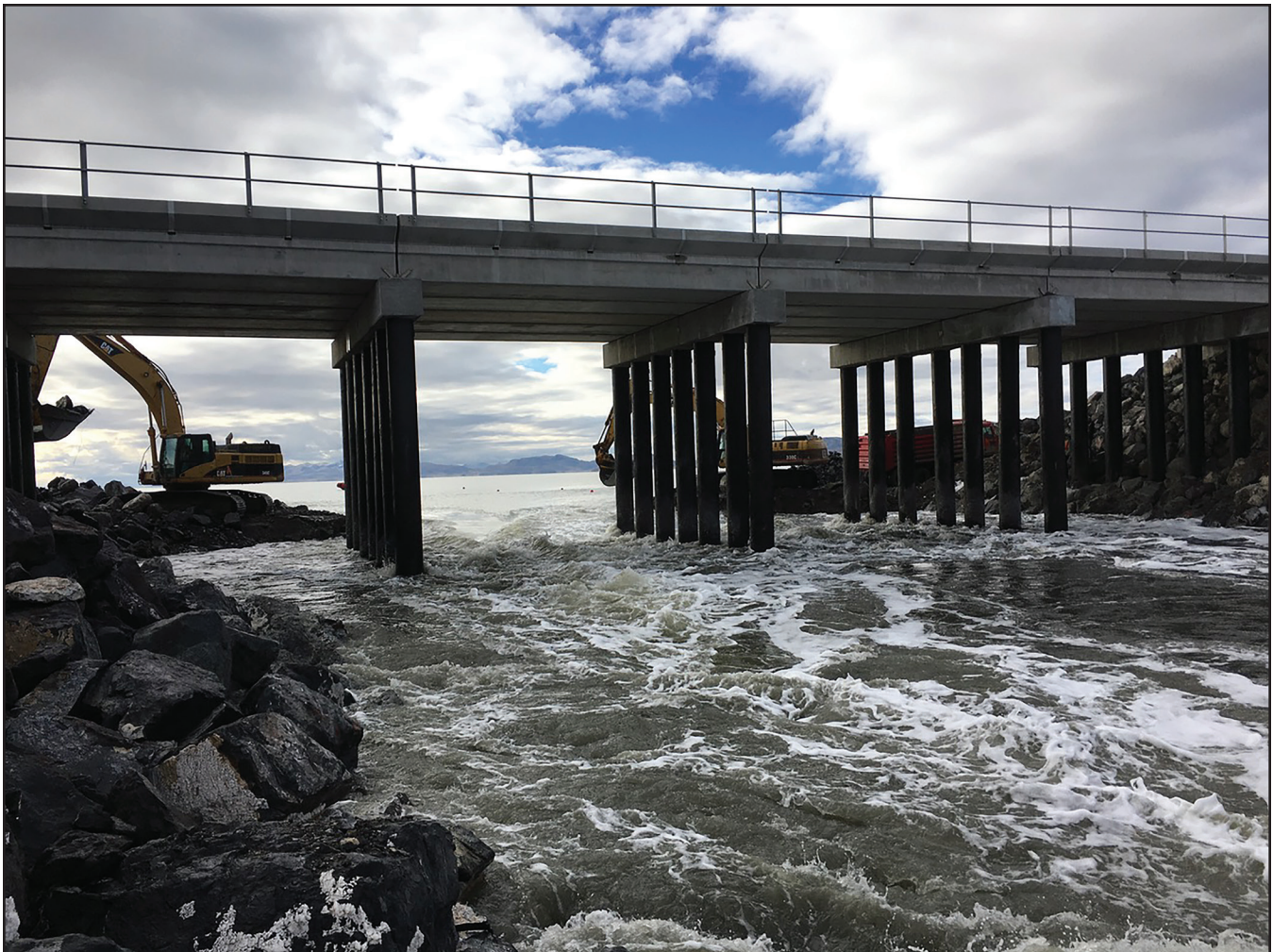
Union Pacific Causeway berm, photograph courtesy of USGS.
